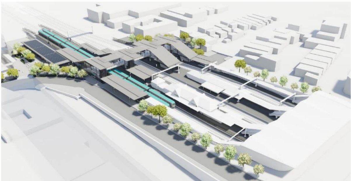
Figure 4.1.4: Aerial view showing integration of photovoltaic roof panels on the northern services building
