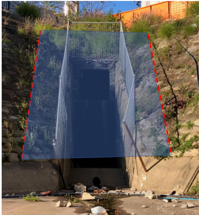
Figure 2. Photograph of Outlet B, with annotations indicating the extent of the proposed modifications to the outlet, and amount of sandstone fabric to be removed.
