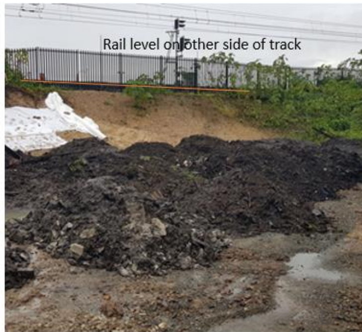
Figure 6: Image of rail line showing introduced fill to build up area of track.
