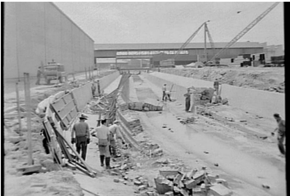
Figure 9 - Storm drain, Sydenham 1965. The image shows the removal and replacement of the c.1898 brick channel by the extant concrete channel adjacent to Sydney Steel Company, looking north (SLNSW Government Printing Office 2 – 26989)
