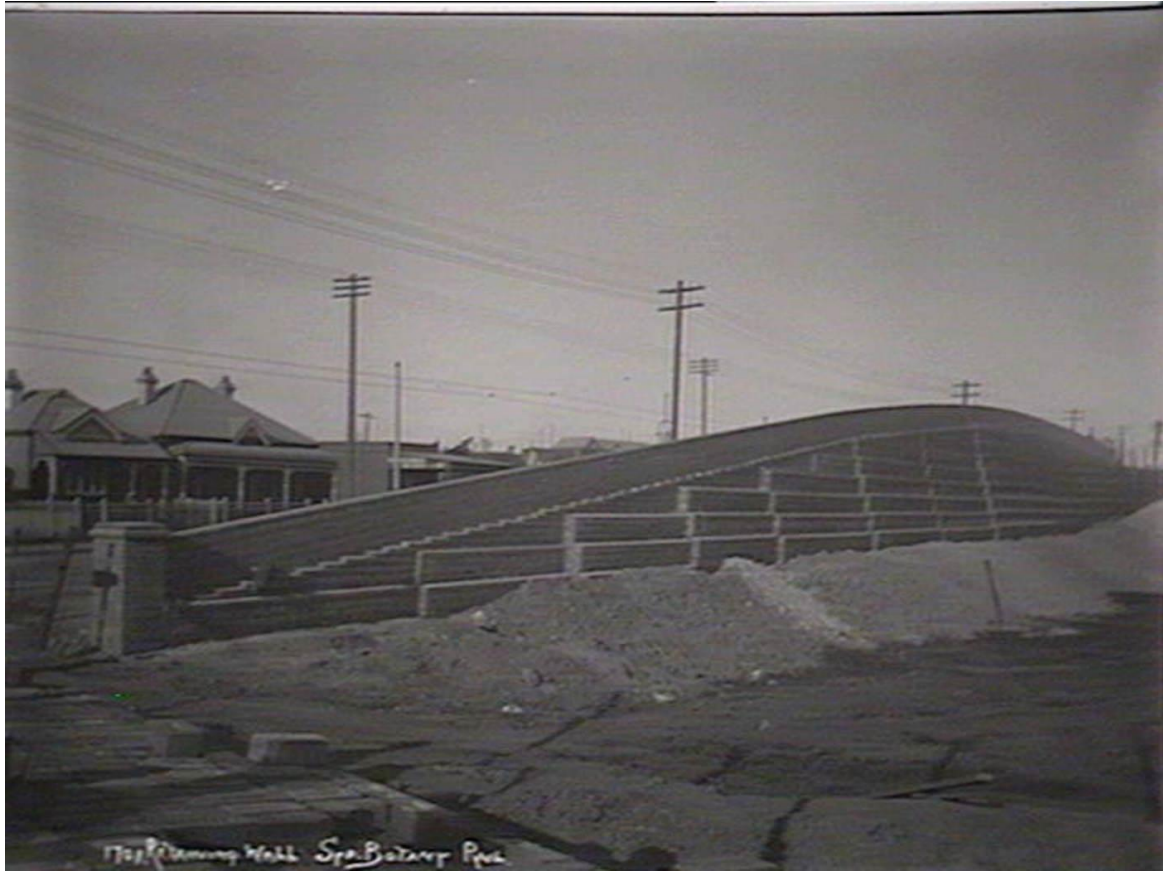
Figure 11 - Construction of retaining wall adjacent to Railway parade, Sydenham n.d. (1916). Looking northwest, the image shows the now-concealed rear of the retaining wall. (SLNSW image 221584)
