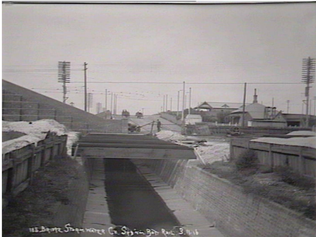
Figure 10 - Bridge, stormwater channel, Sydenham - Botany rail, 3 November 1916. View shows the 1898 stormwater channel, the Marrickville Road railway embankment wall (left), the Sydenham station concourse buildings (top right) and the buildings that occupied th
