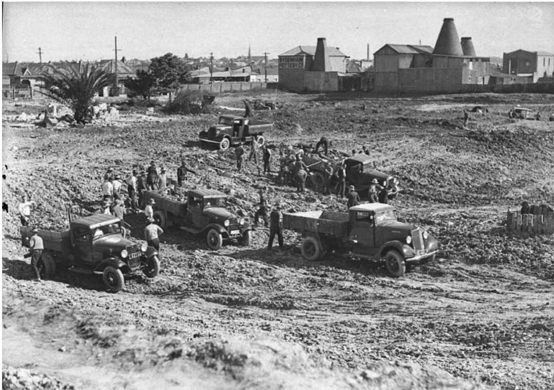
Figure 8 - Works at Sydenham 1935 (SLNSW 81937). Excavation of the Sydenham Drainage Pit looking northwest towards the Garden Street/Shirlow Street intersection. The Sydenham Pottery Company at top right.
