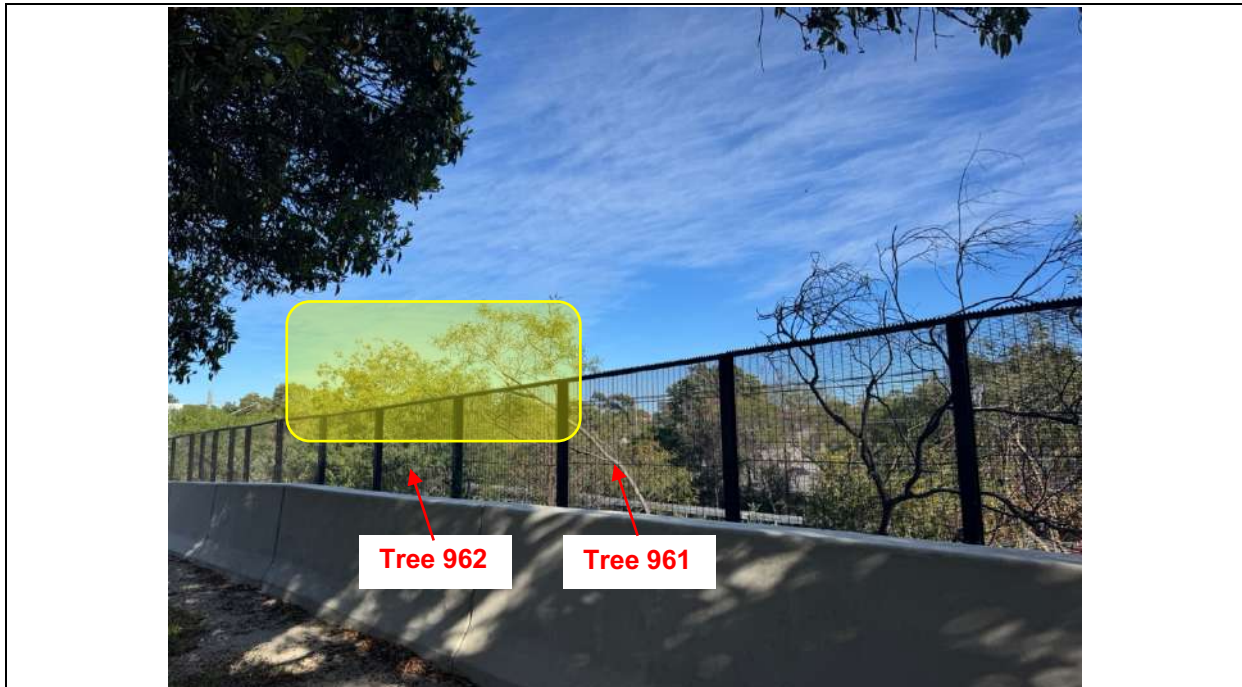
Image 8: Looking towards trees 961 and 962. Canopy pruning is required to provide 2m clearance from the fence. Smaller branches measuring less than 50mm in diameter are to be pruned. The pruning will result in the removal of 10% of the live foliage area of each tree.
