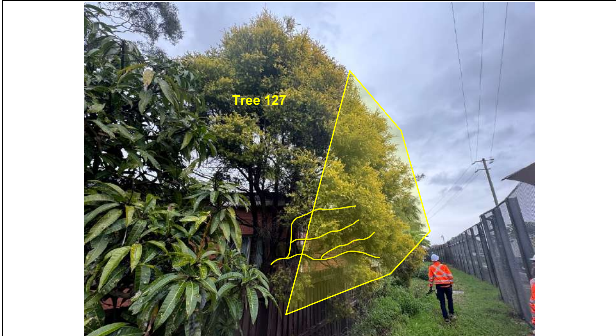
Image 2: Looking towards tree 127, showing the area of foliage requiring pruning. The low 130mm diameter branch towards the corridor is to be removed, and additional smaller branches towards the corridor that measure less than 30mm are to be removed. Approximately 30% of the live foliage area will be removed.
