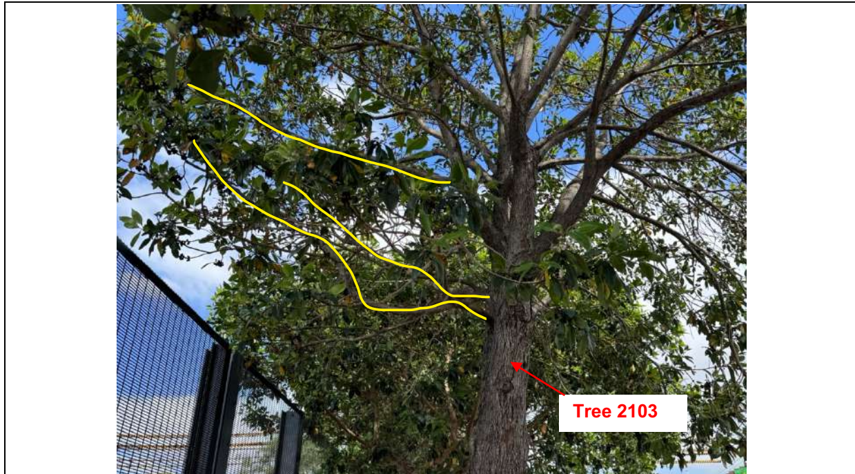
Image 27: Looking towards tree 2103. The three branches marked yellow require pruning to provide fence clearance. The pruning will result in the removal of approximately 5% of the live foliage area of the tree. The maximum finished cut diameter measure less than 60mm
