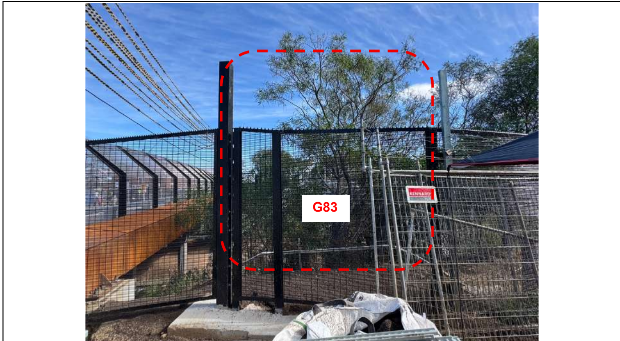
Image 15: Looking towards tree G83, which is a group of five trees. The trees are recommended for removal.
