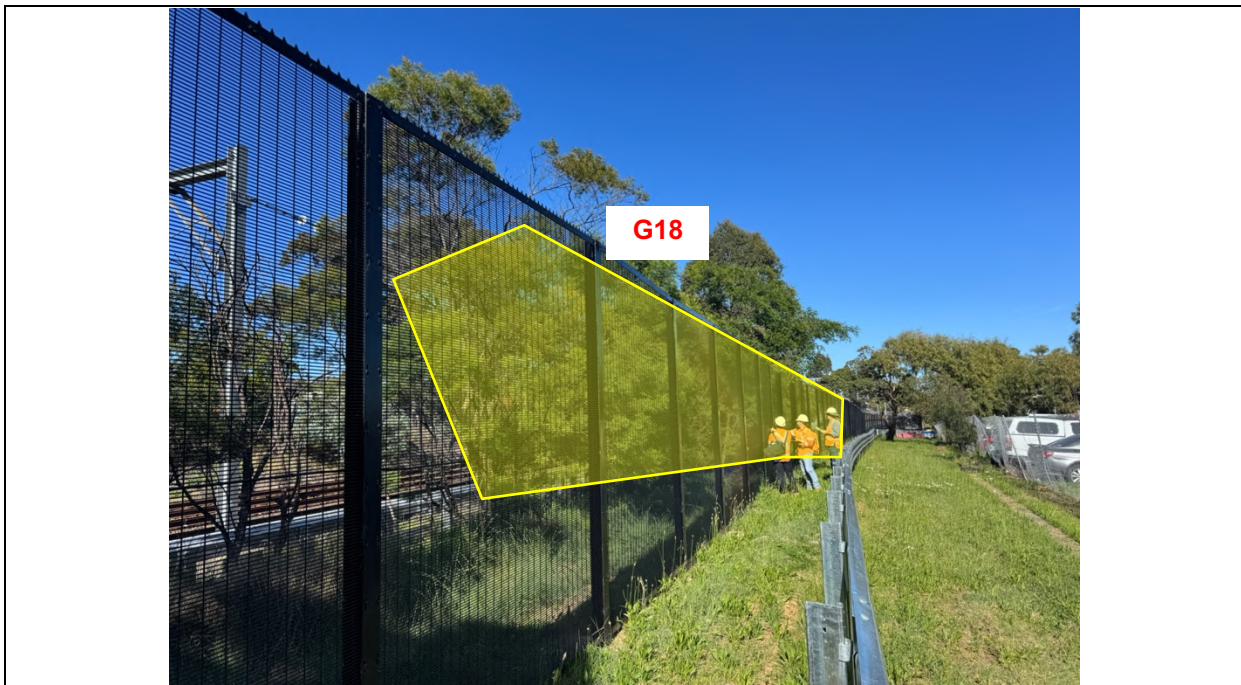
Image 12: Looking towards G18, which is a group of approximately 46 trees recommended for pruning. Smaller branches measuring less than 50mm in diameter are to be pruned. The pruning will result in the removal of less than 10% of the live foliage area of each tree within the group. The approximate area of the pruning has been marked yellow.
