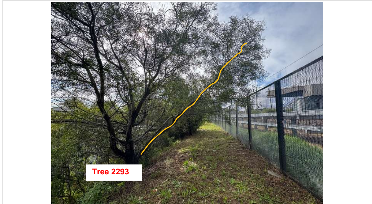
Image 21: Looking towards tree 2293. Canopy pruning is required to provide 2m clearance from the fence. The first order branch to the South (finished cut diameter of 180mm) is to be removed. The pruning will result in the removal of approximately 15% of the live foliage area of the tree. The branch to be removed has been marked yellow.
