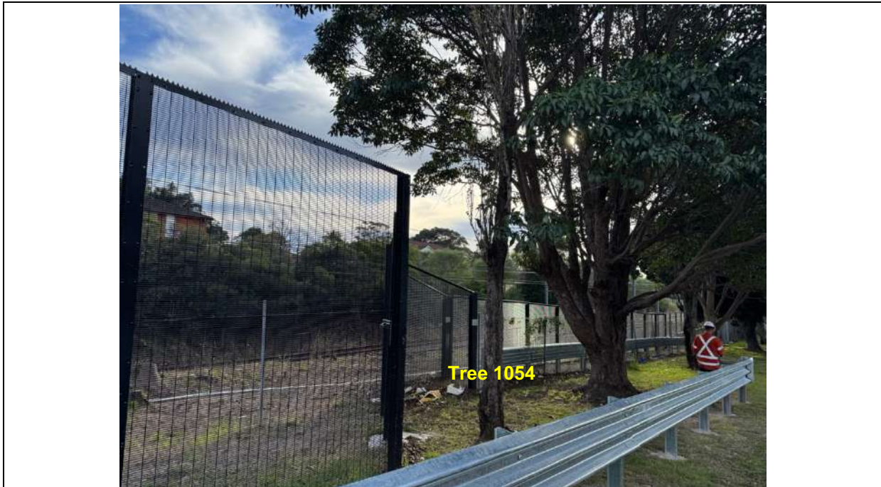
Image 21: Looking towards tree 1054. The tree is recommended for removal for fence clearance requirements.
