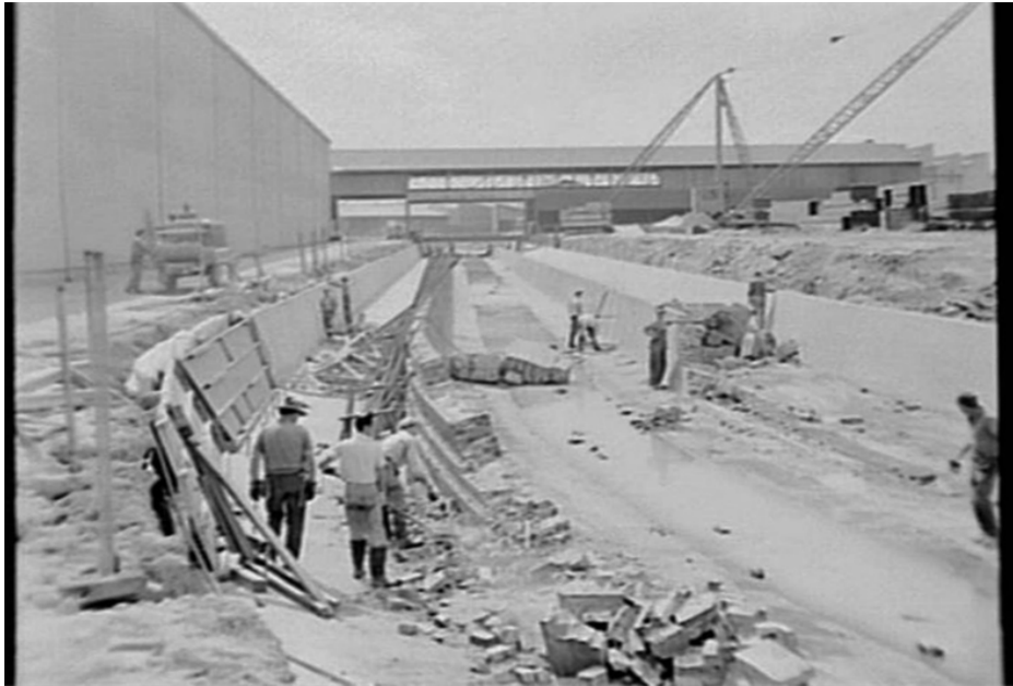
Figure 24 Storm drain, Sydenham 1965.
