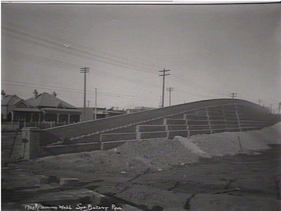
Figure 26 Construction of retaining wall adjacent to Railway parade, Sydenham n.d. (1916).
