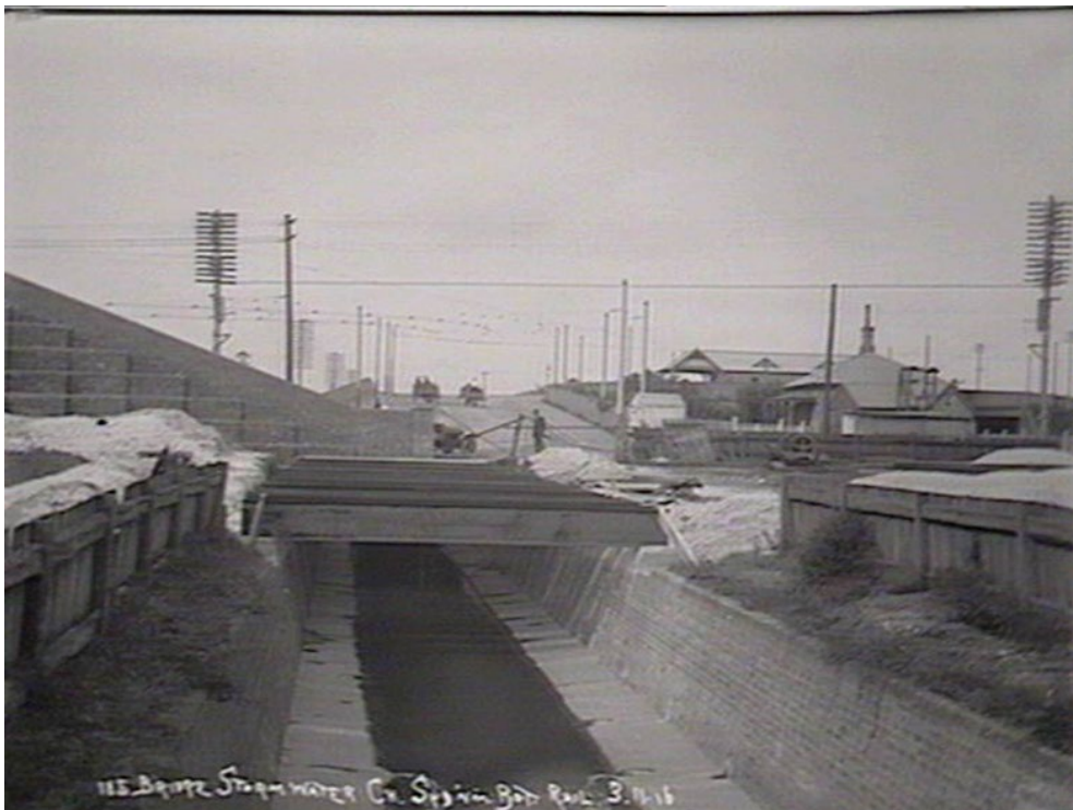
Figure 25 Bridge, stormwater channel, Sydenham - Botany rail, 3 November 1916.
